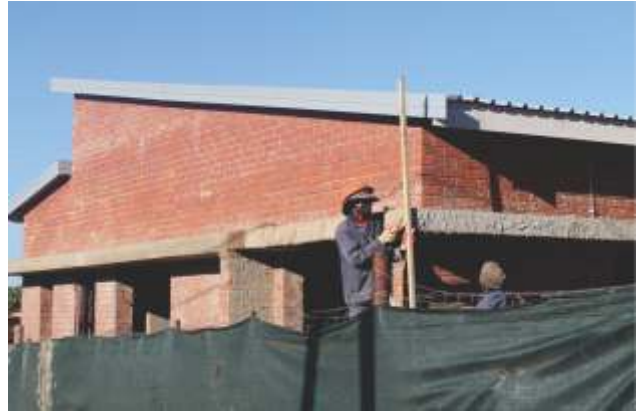
The construction work on the project created 62 work opportunities for both professional and general labour.
