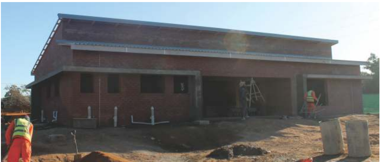
The Daggakraal ECD Centre currently under construction.
